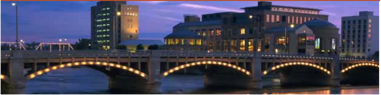
Lighted Bridge on the Grand River. Photo: Brian Kelly. Courtesy Grand Rapids/Kent County Convention and Visitors Bureau
